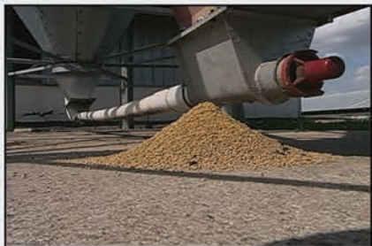
Eliminate all spilled feed
