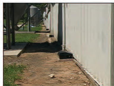
Keep a 3-foot sterile zone around buildings mowed or sprayed
